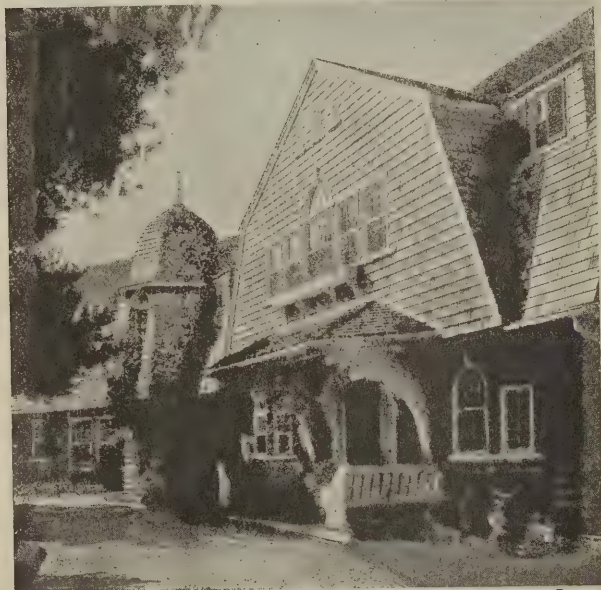
TYPE OF STRUCTURAL WINDOW BOX. WOULD BE BETTER IF EXTENDED THE WHOLE WIDTH OF THE SPACE UNDER THE WINDOWS
